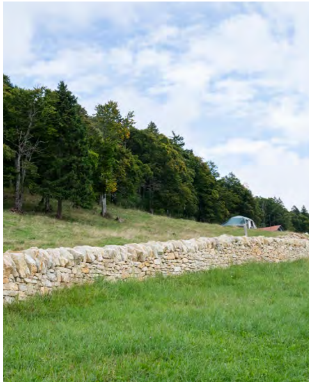
The dry-stone wall on Grenchenberg is rising up again.
