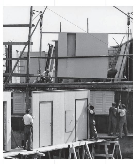
Göhner building constructed using prefab elements, 1950s
